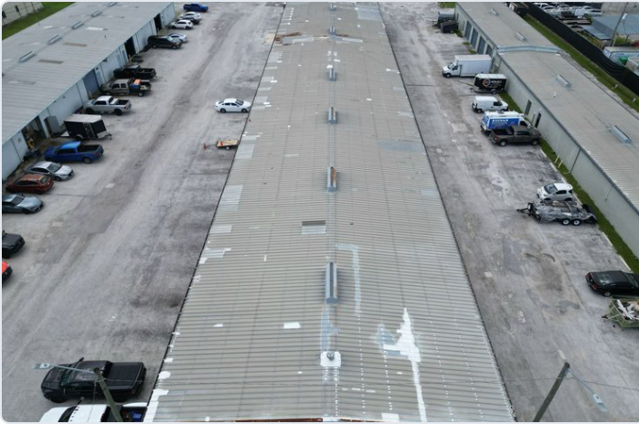
05 Overall view of the B roof — 18,561 SF of PBR panel. White silicone repairs are distributed across the full length of both slopes.
